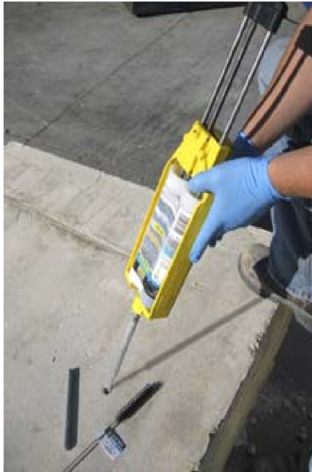
Figure 1: Adhesive delivery using a mixing nozzle and dispensing tool.
