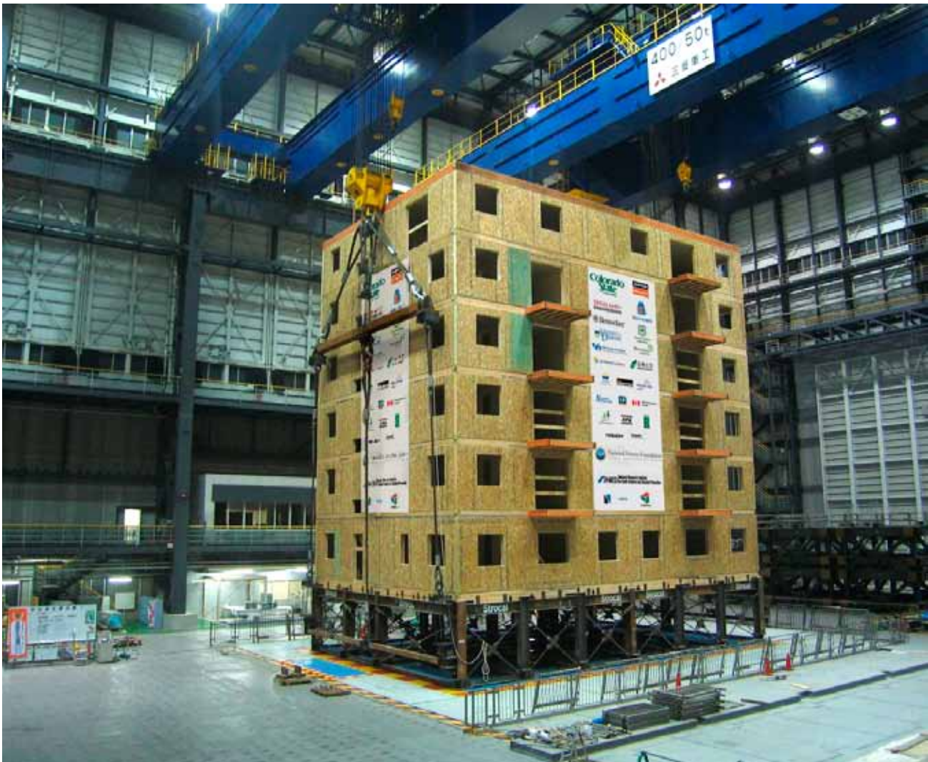
A full-scale, seven-story, wood-framed condominium tower – secured with Simpson Strong-Tie® products, including steel special moment frames and 63 Anchor Tiedown System runs and structural connectors – withstood a 7.5 magnitude simulated earthquake with only minor drywall damage in the world's largest earthquake shake table test. The 2009 NEESWood Capstone project was developed to test new design methods for multi-story, wood-frame buildings during large seismic events, and highlight the importance of earthquake-resistant construction around the world.
