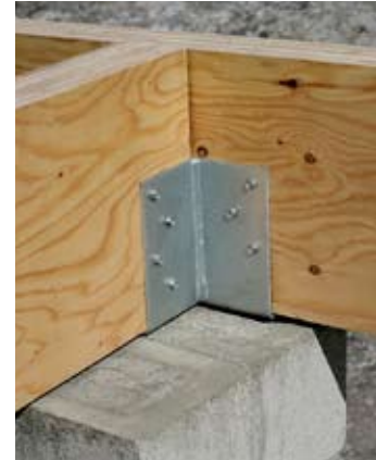
Typical CCTQM Installation
