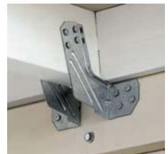
Typical HPTSS installation
