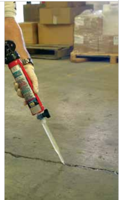
Crack-Pac® adhesive gravity-fed into horizontal cracks
