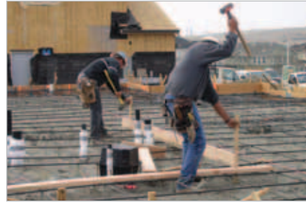
Setting interior forms requires precise placement and extra labor.
