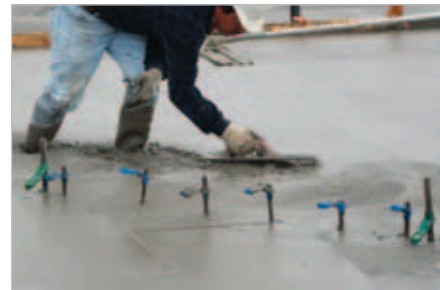
Removing interior forms, adjusting anchors and refinishing slows down the pour.
