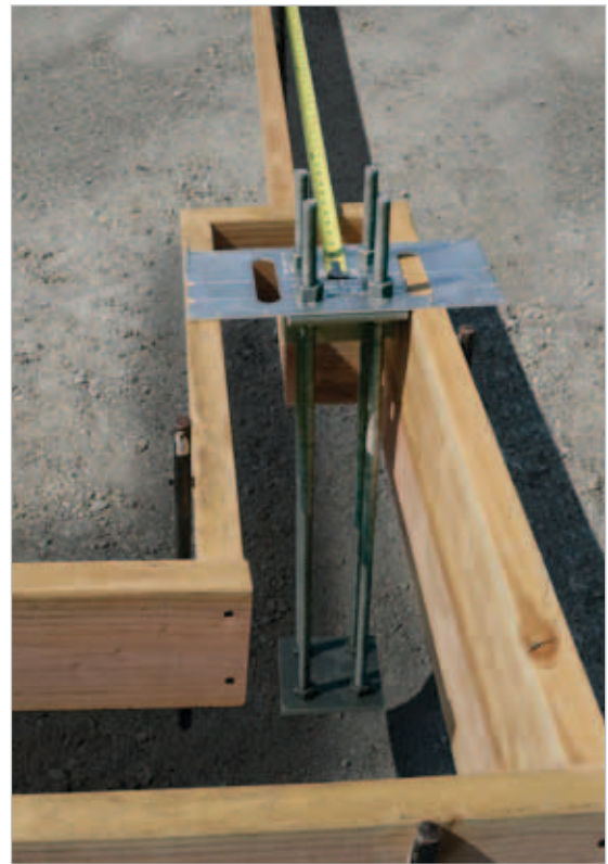
Strong Frame™ OMFSL anchorage assemblies make design and installation faster and easier.
