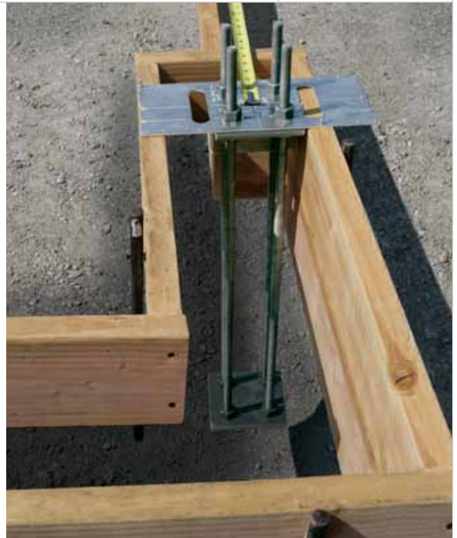
Strong Frame™ OMFSL anchorage assemblies make design and installation faster and easier.
