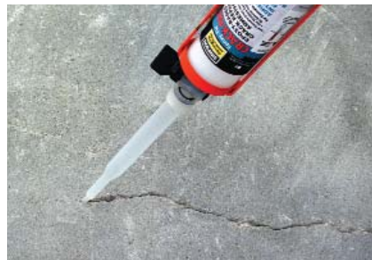
ETI and Crack-Pac are ideal for repairing cracks in concrete slabs.
