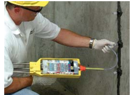
The dual cartridge system makes the ETI epoxy simple to use.
