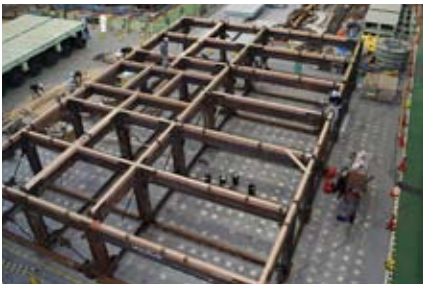
Special Moment Frames are constructed on the first level.
