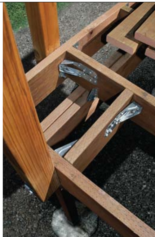
Guardrail-Post Connection
