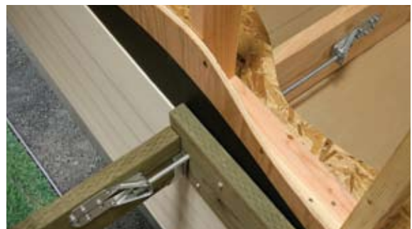
Deck-to-House Lateral-Load Connection
