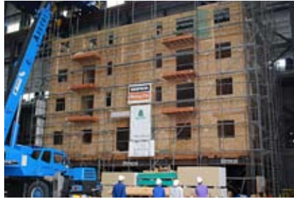
Carpenters continue to work on the 7-story structure.
