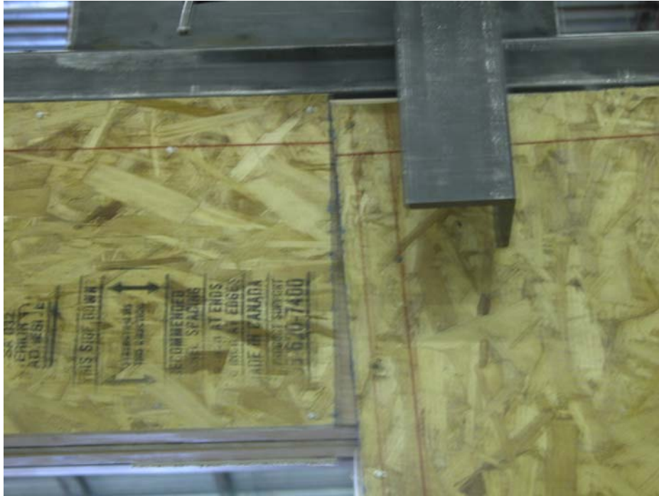
Figure 9. Secondary Failure of 4_1 Wall Frame Specimens – Separation and Cracking of OSB.
