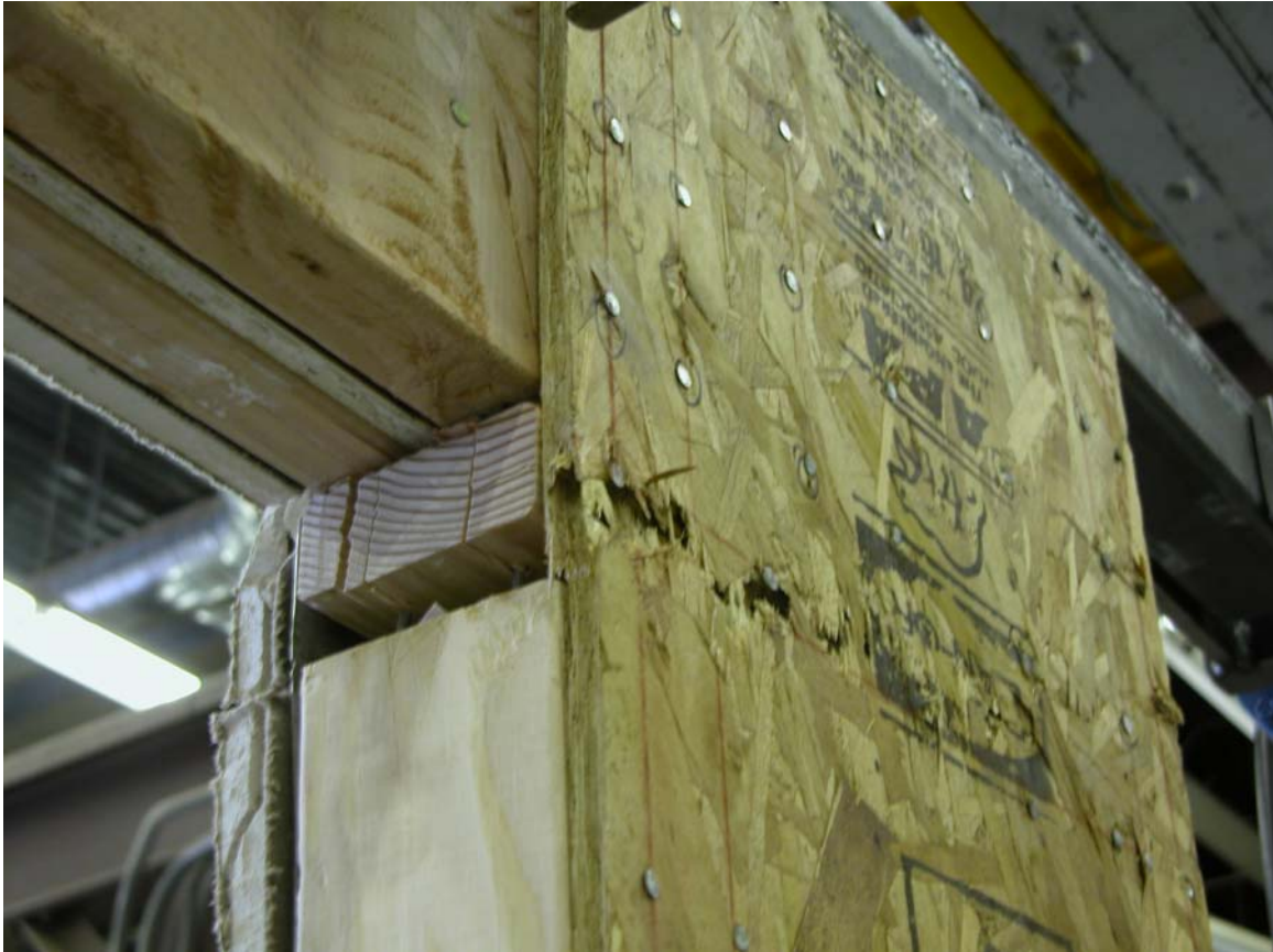
Figure 5. Secondary Failure of Portal Frame Specimens – Cracking of OSB.
