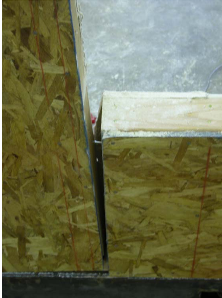
Figure 11. Continued Failure of 4_1 Wall Frame Specimens – Separation of Wall Segments.
