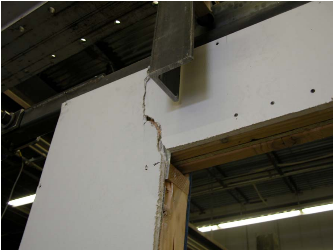
Figure 4. Typical Initial Failure of Portal Frame Specimens – Cracking of Gypsum Wallboard.
