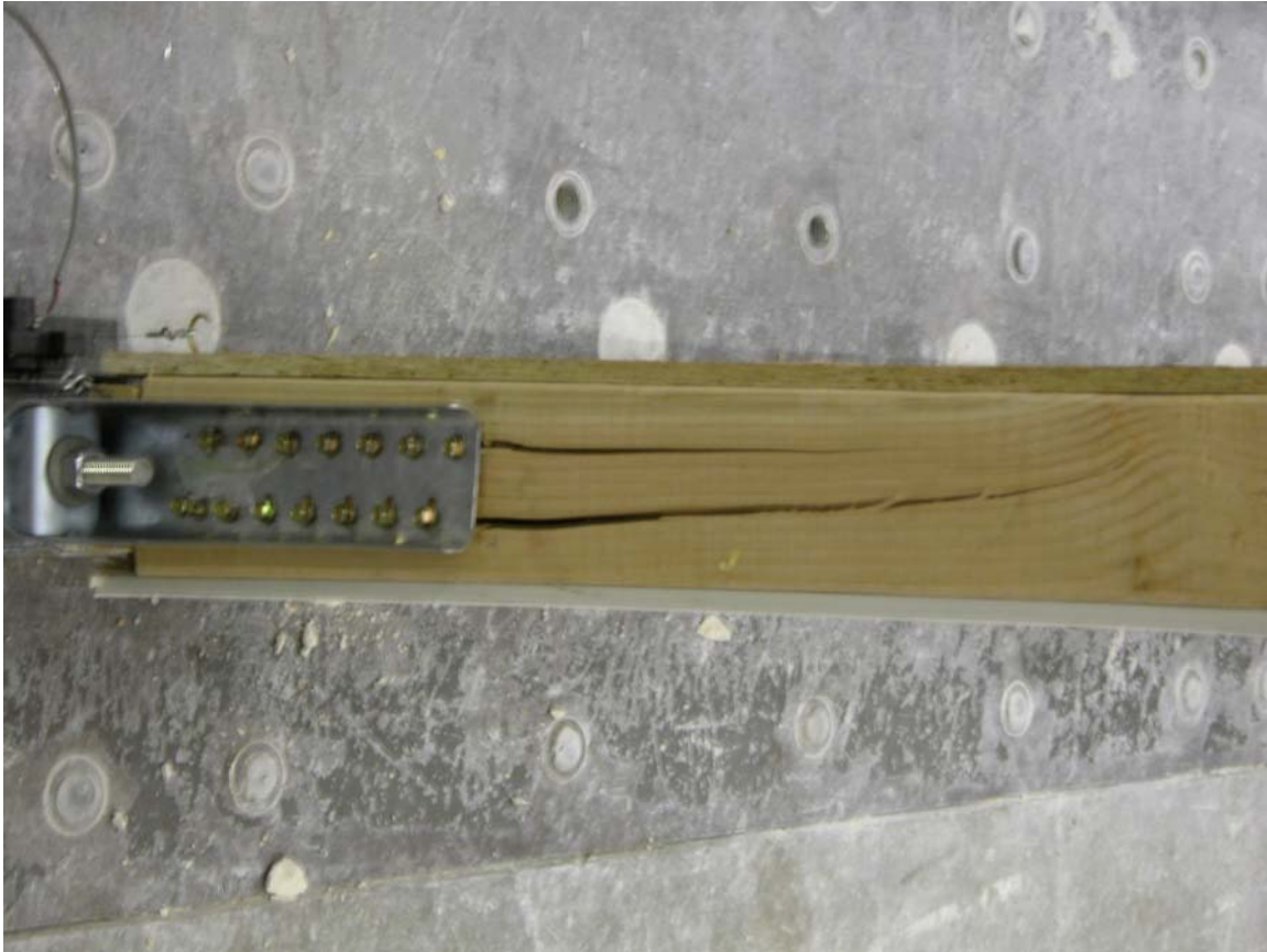
Figure 7. Typical Failure of Hold-Down Post – Occurred at Large Displacements.
